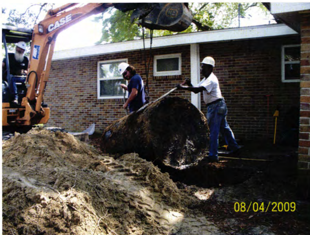
Picture 2: UST 1438Dove.
