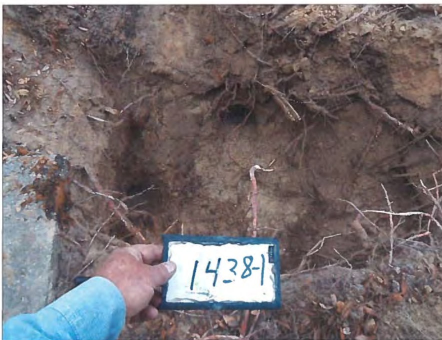
Picture 2: UST 1438Dove-1 excavation.
